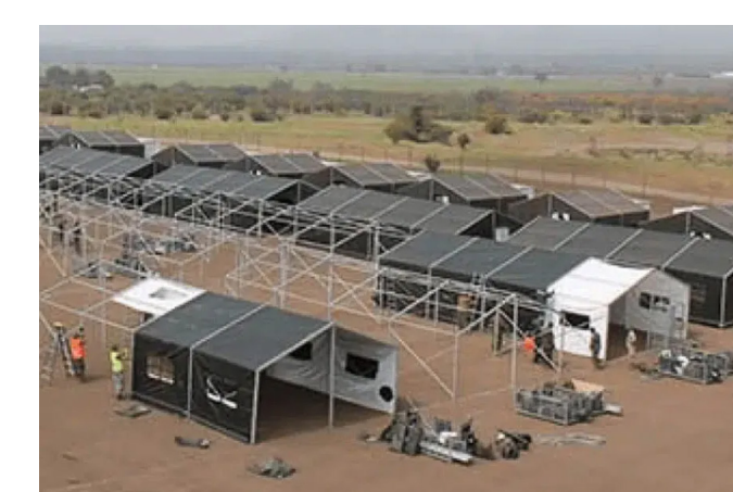
Post-disaster relief tents being constructed
